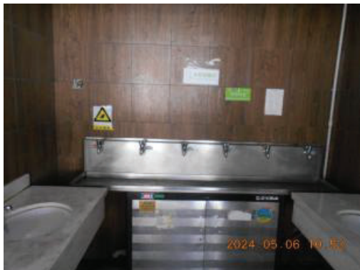
Drinking water facility.JPG
