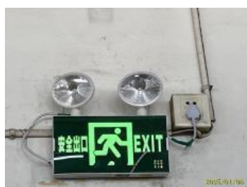
Safety exit sign and emergency light.JPG
